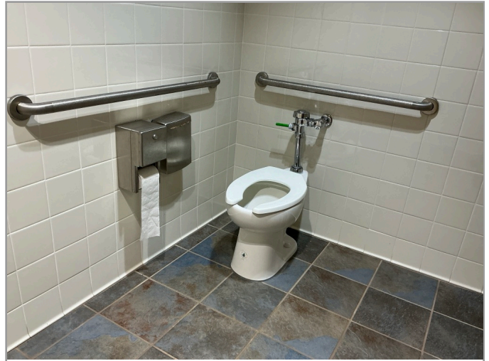
TOILET STALL OVERVIEW
