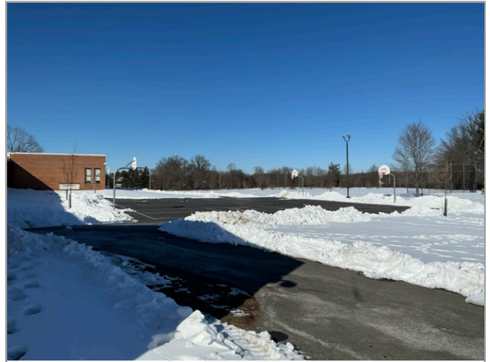
ACCESSIBLE ROUTE TO PLAYGROUND
