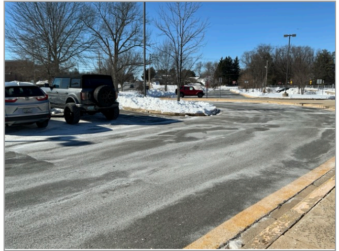
OVERVIEW OF ACCESSIBLE PARKING AREA
